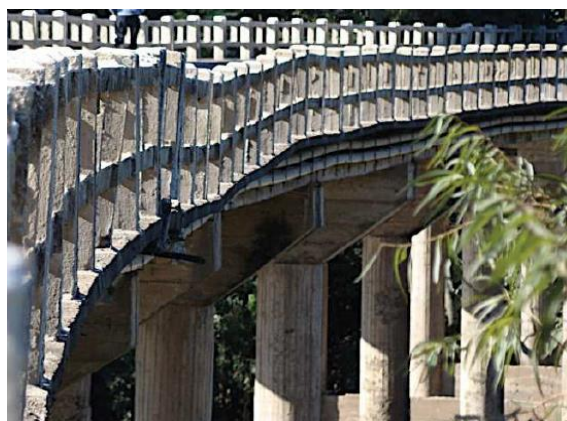
Figura 22: recalque ( F_i = 4 )
