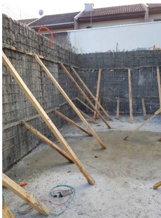
Figura 17 – Chapisco no painel (Calure Engenharia, 2019)
