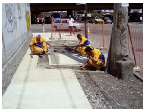
FIGURA 2.11 – Moldada in loco .
