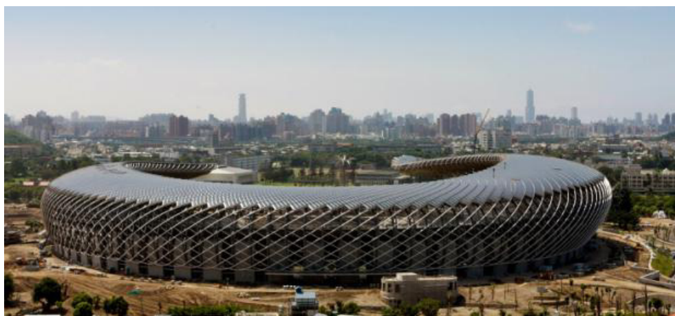
Figura 12 – Fachada do World Games Stadium
